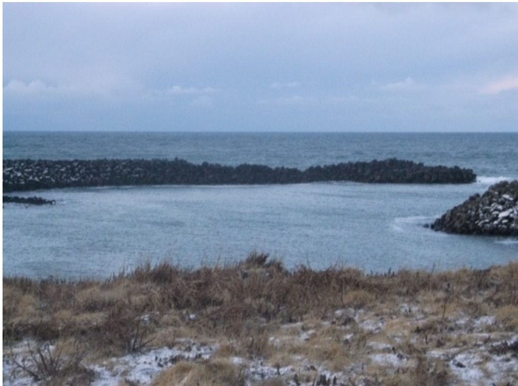
Figure 7: View of Same Portion of South Breakwater from a Different Angle. Material missing from the breakwater is evident.
